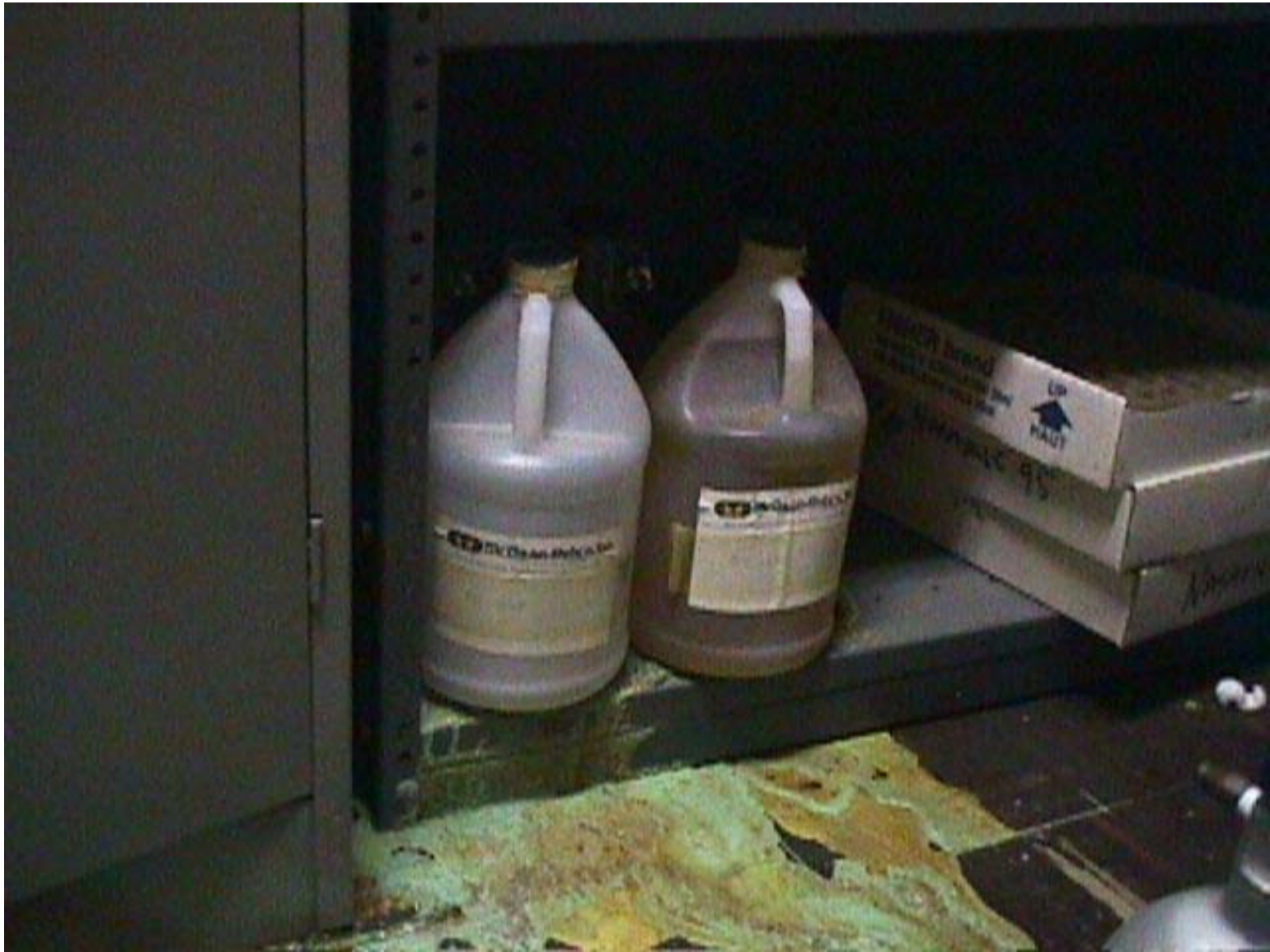
Damage from leaking chemical
